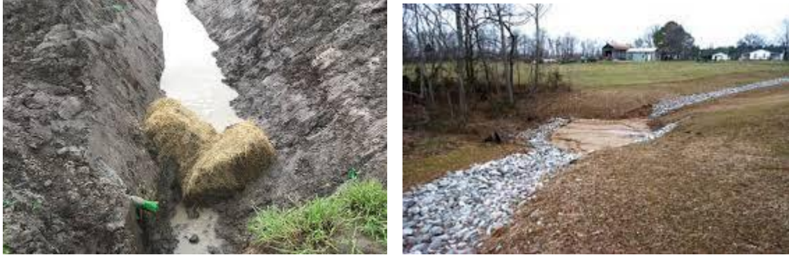
Figure 8: Typical Diversion Drain Installations
