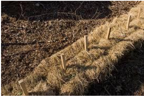
Figure 6: Typical Straw Bale Installations
