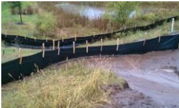
Figure 7: Typical Silt Fencing Installations
